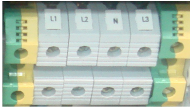
Photo 13 : Disposition borniers.
